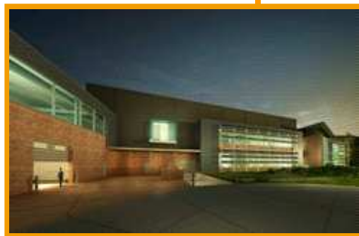
Stony Brook University AERTC Building
