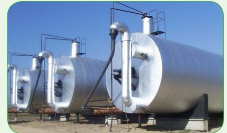
A biogas digester separates animal waste into manure and valuable methane
