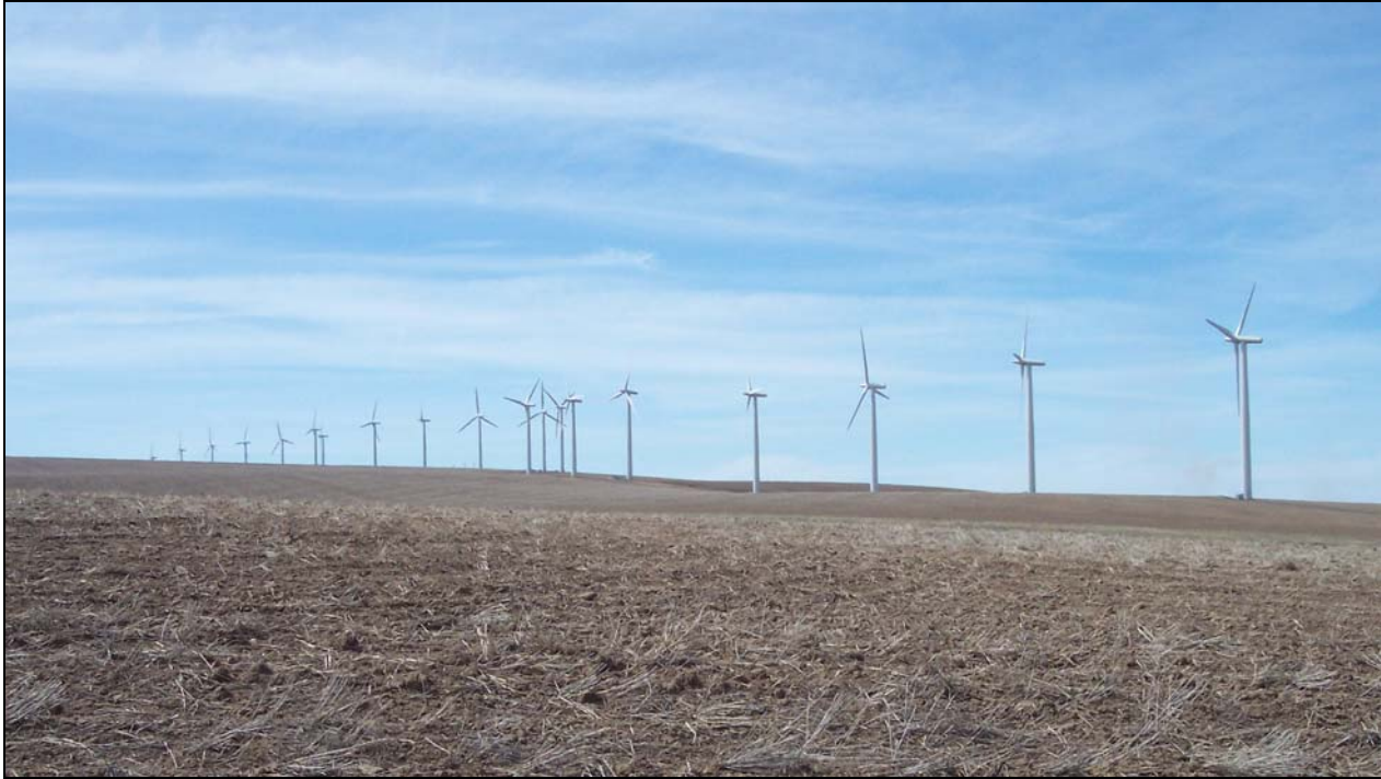
49 x 1.3 Mw, WIND FARM INTEGRATED INTO HYDROELECTRIC POWER SYSTEM / WASHINGTON STATE, USA PHOTO CREDIT: LARRY FELTON, FELTON AND ASSOCIATES.
